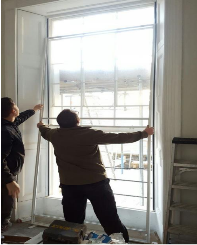
Installing slimline secondary glazing
