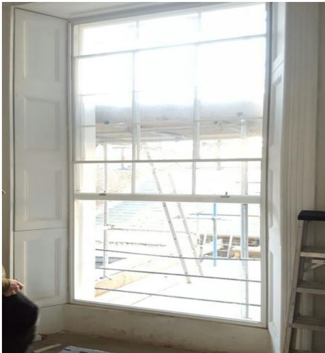
Installed slimline secondary glazing
